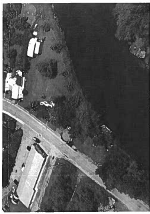
View of the bridge abutments
